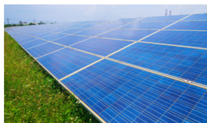
Solar Cell Inspection
